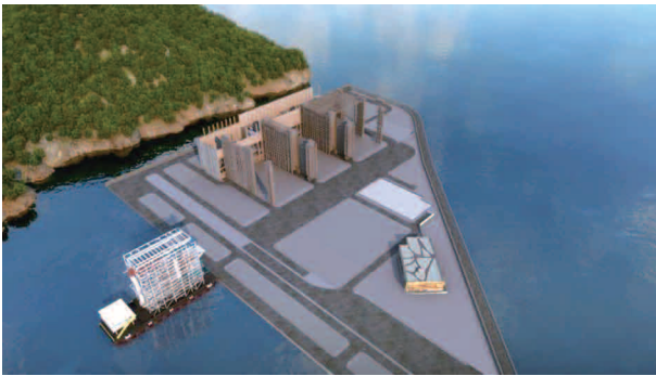
Figure 5 - Prefabrication Boiler Module deliver simulation for programme planning and construction sequence design.
